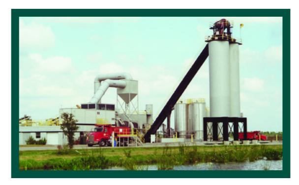
An asphalt plant is where materials are brought together and blended into Hot Mix Asphalt, which is transported to the paving site for construction into a pavement.
